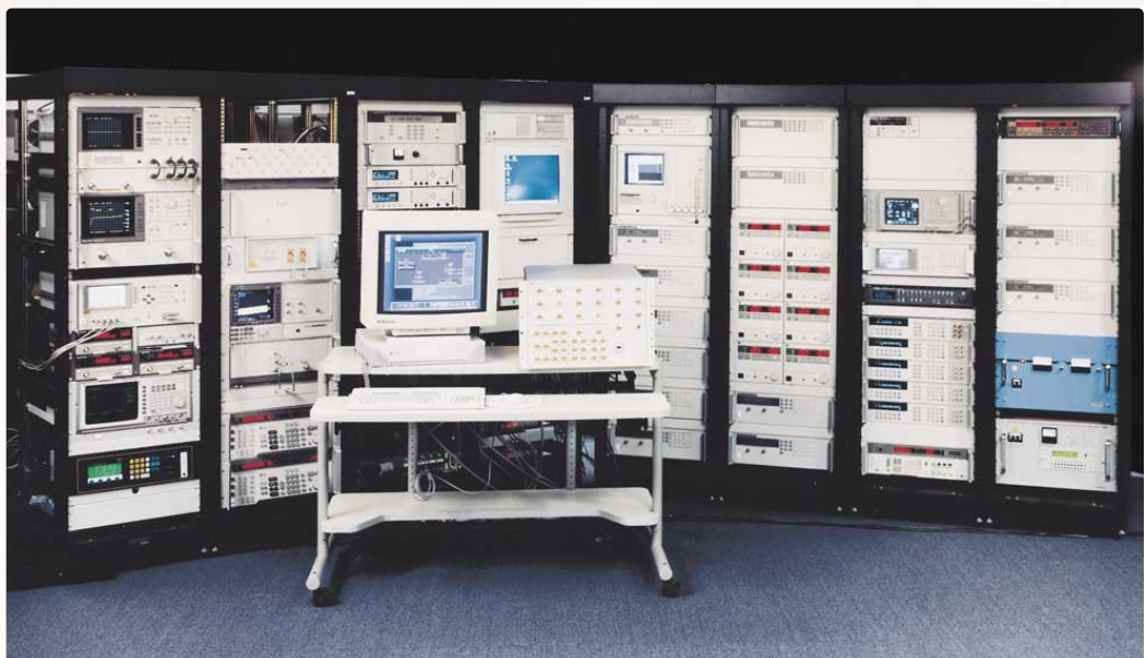
B2 avionics test bay subsystem
